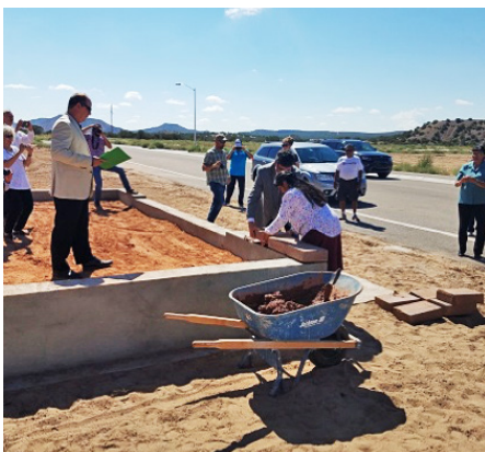
As part of one DEMD contract, Flatwater Group worked with mineral geologist Amanda Irons in New Mexico to formulate high-performance adobe bricks and plaster. The homebuilding materials are made from locally available resources such as pumice stone, gravel or sand. This benefits the community's sustainable housing efforts and local economy.
